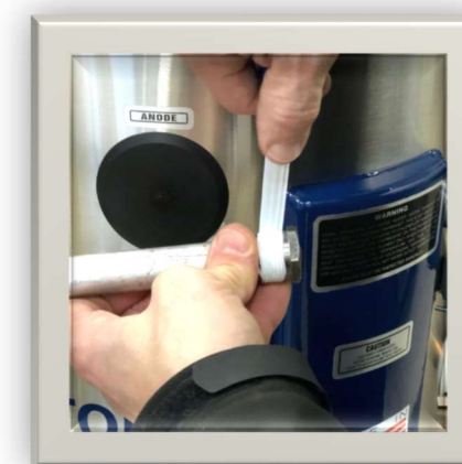
Image 1.3 Install new anode with PTEF tape or sealant.
