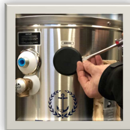
Image 1.1 Locate anode and remove plastic cover.
