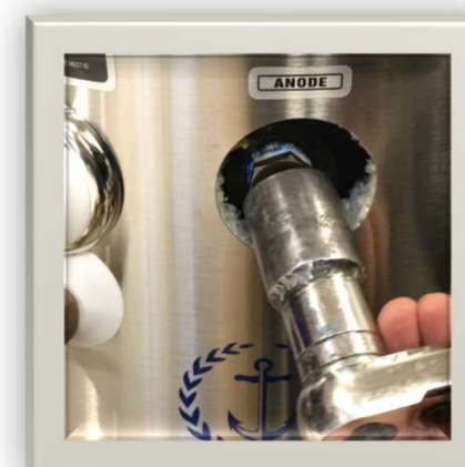
Image 1.2 Remove anode with 1-1/16" socket.
