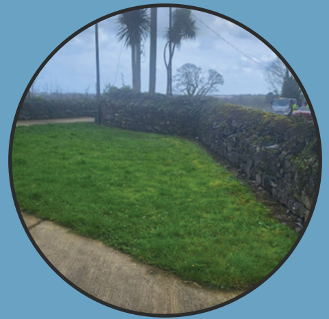
Areas around Carlingford Castle are perfect areas to be managed as wildflower meadows.
