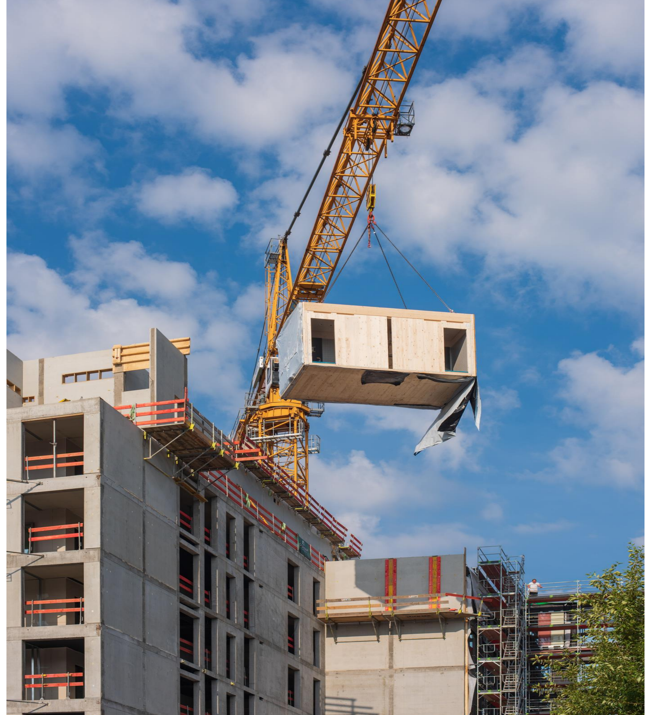
Image: Modular construction unit being lifted into place. Licensed stock image purchased by the editor, 19 May 2026.
