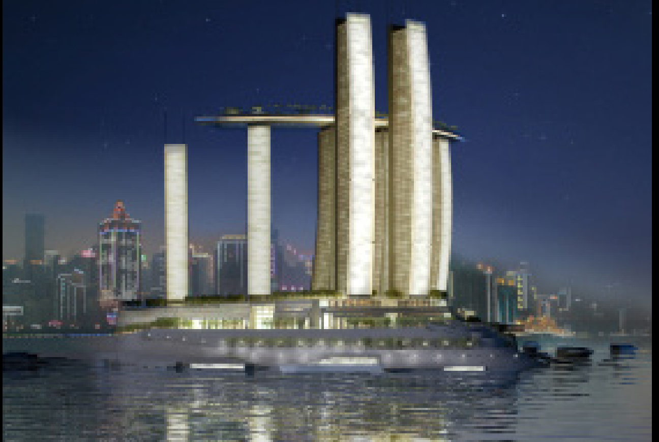
Final Competition model Dynasty Raffles City Chongqing, China 1-200 scale Foam, acrylic and PETG base, solid massing buildings - basswood, light buildings- painted and clear lasercut PETG.
