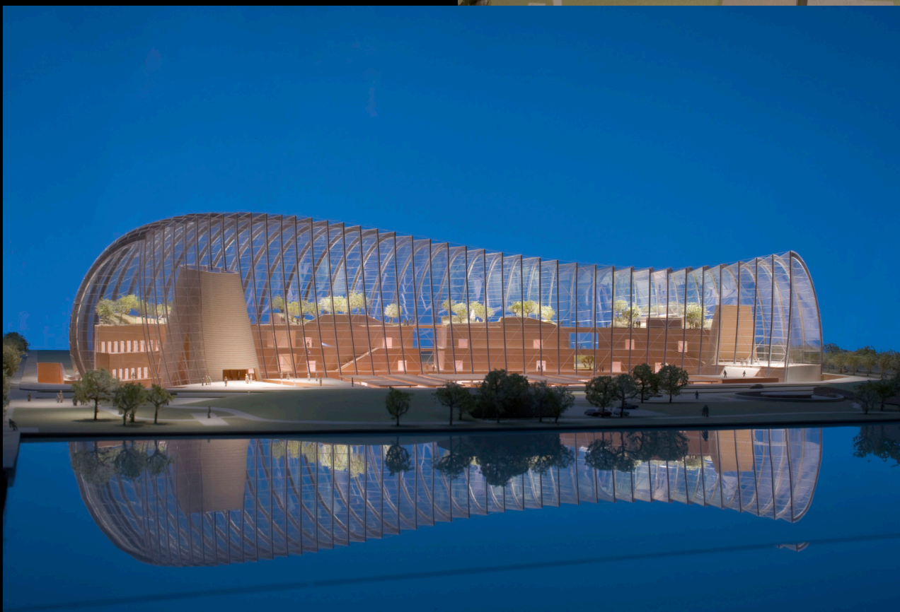
Final Competition model National Art Museum of China China 1-200 scale Foam, acrylic block and PETG base, interior buildings - solid acrylic clad in basswood veener, shell - painted and clear lasercut PETG.
