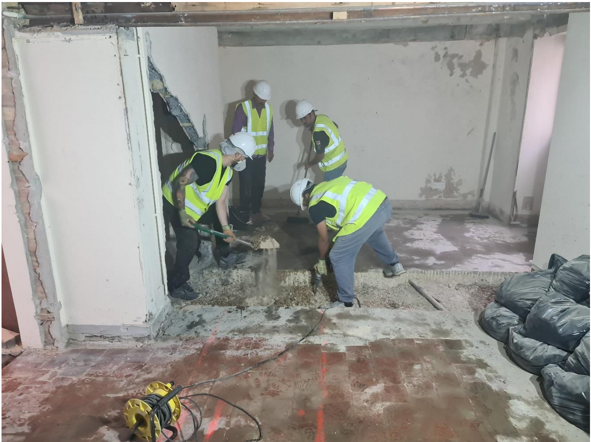
Plate 3 Hand excavation of the foundation trench
