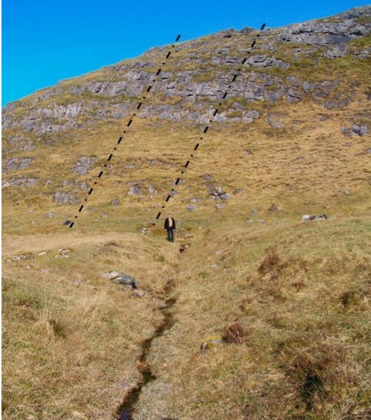
Figure 10. The lade leading towards the mill from Loch Borralie. The faults in the limestone ridge into which the stream disappears are shown as broken black lines. The upper house is located at the far end, to the left of the person.
