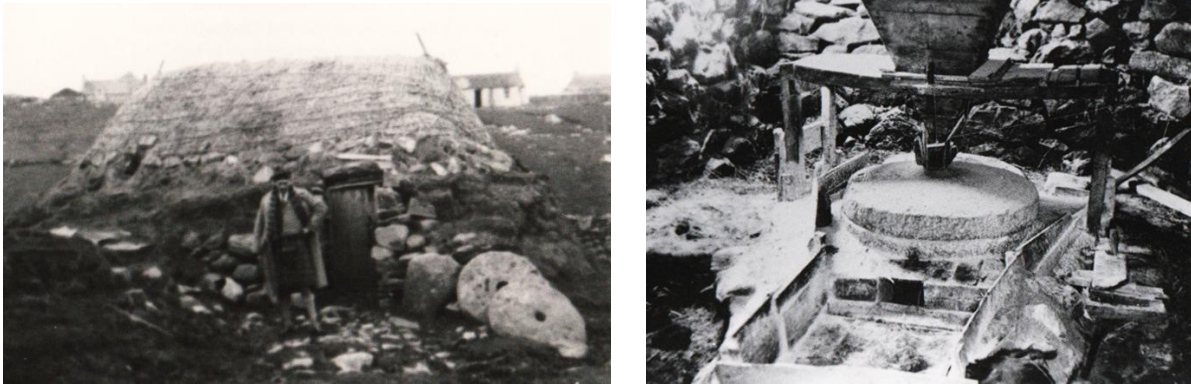
Figure 1. The Norse mills did not always have to be sophisticated (left photo) as long as they served their purpose (right photo). These photos are of working horizontal mills on the Isle Lewis from 1930 and 1935 respectively (Macleod, 2009).
