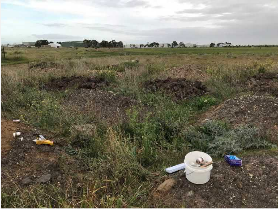
Plate 13: Surface condition of stockpiles along southern boundary ; at STP12, facing north-west.
