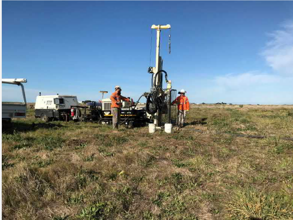
Plate 15: Groundwater well installation at MW001
