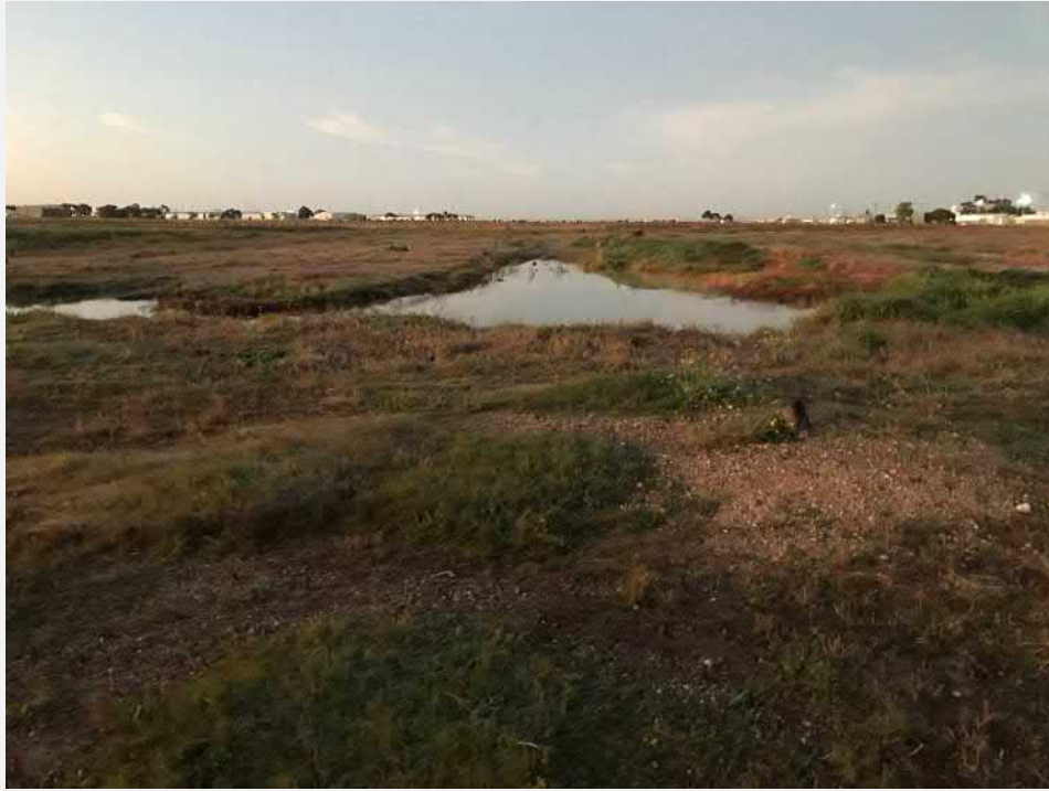
Plate 3: Observed standing water; from HA04, facing south.
