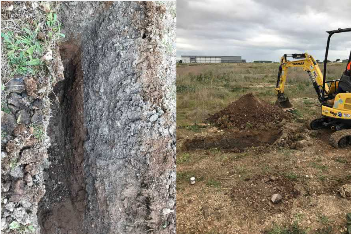
Plate 5: Test Pitting at TP03 and the observed soil profile.
