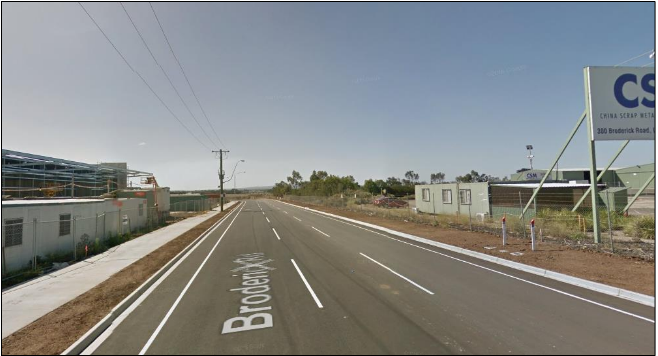
Figure 2-8: Broderick Road south of Production Way intersection looking northbound (Source: Google Street View, 2020)
