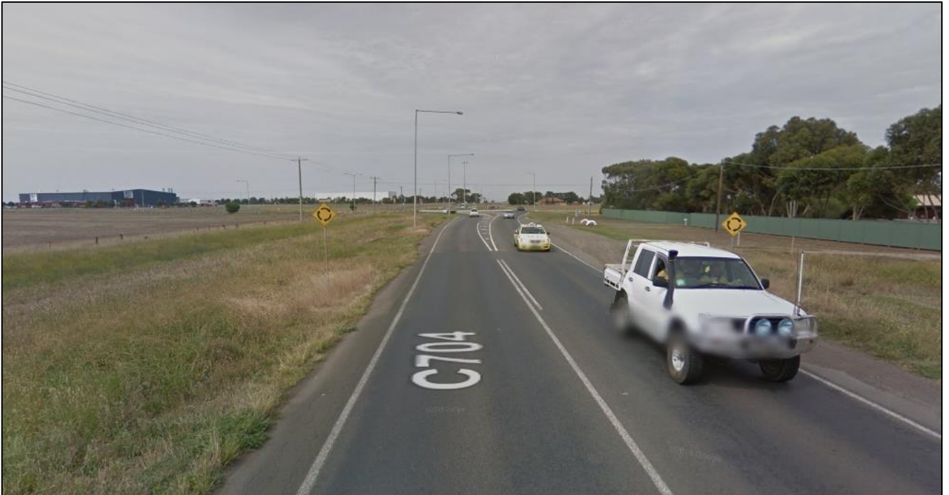
Figure 2-3: Bacchus Marsh Road north of Heales Road intersection looking southbound (Source: Google Street View, 2020)
