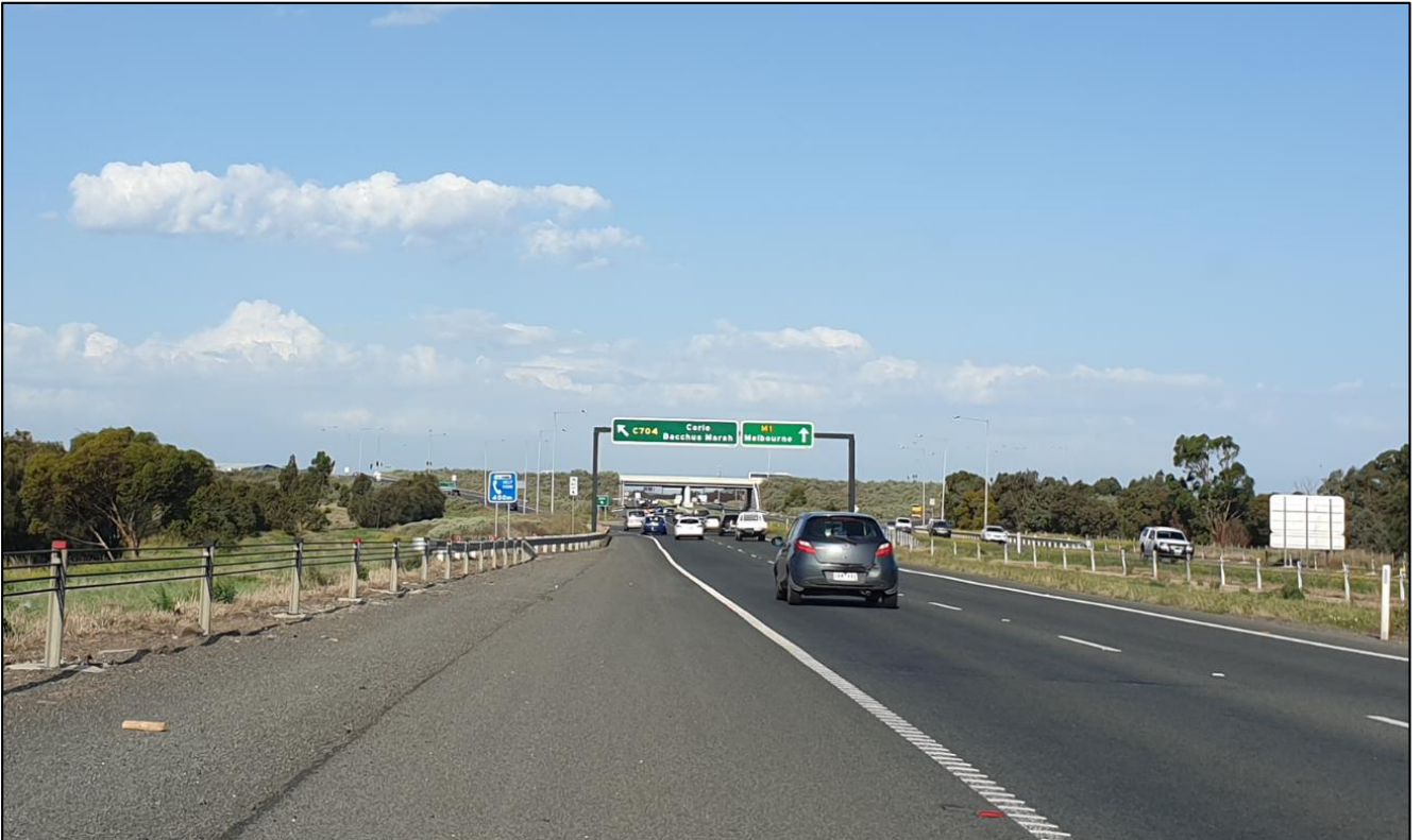
Figure 2-2: View of Geelong Ring Road
