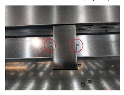
4. Unscrew two screws of conduit remove the cover and slip off the corrugated pipe (see picture)
