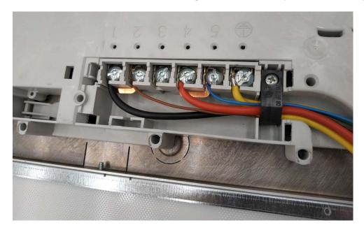
6.3 Remove the induction module and put new one . Fix with the screws around frame . (see picture) . Please take care to insert n . 2 bridge as in the picture at 6.2 .
