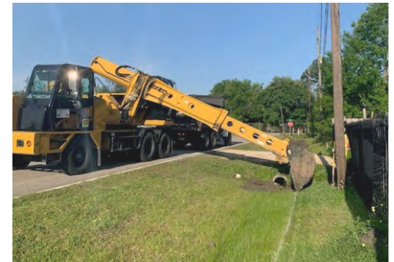
Figure 2.1.14 Ditch Cleaning/Vactoring
