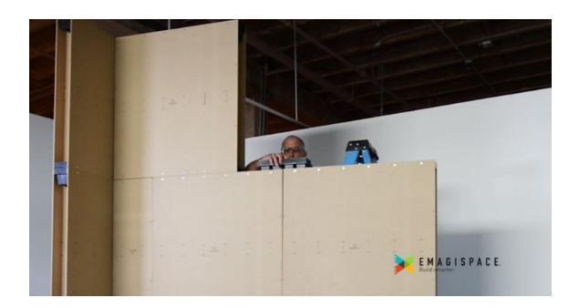
16) Add a 36" EmagiBlock<sup>®</sup> perpendicular to the first course of the wall. This will be the second support wall.
