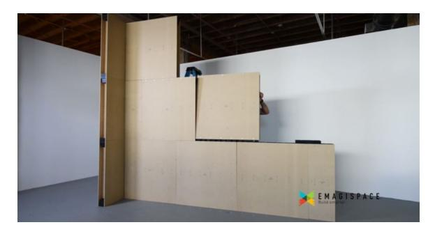
15) Use a Block Connector to temporarily secure this 36" EmagiBlock  $^{\circledR}$  to the second course.
