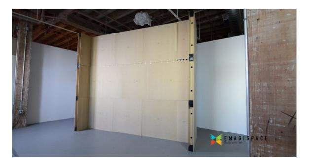
26) Secure the 12" EmagiBlock<sup>®</sup> to the second support wall and ensure that all EmagiBlock<sup>®</sup>s on the third course are secured to each other with connector blocks. Secure the EmagiBlock<sup>®</sup> to the wall by screwing through the two screw holes in the connector block (screw directly into a stud when possible)
