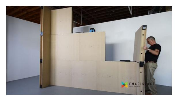
18) Secure the first course of the wall to the support wall, by screwing through the two screw holes in the connector block (screw directly into a stud when possible. If not possible, use toggle bolts / plate and/or other industry standard methods to insure stability.)
