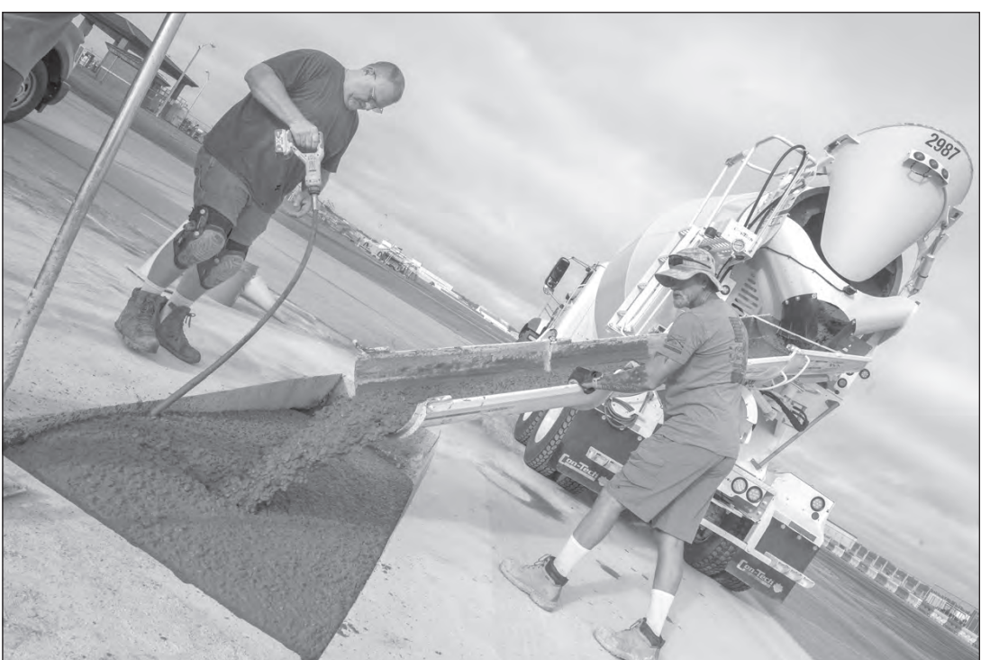
Robert Wreden, right, 78th Civil Engineer Squadron mason, directs concrete flow into a taxiway repair hole while Travis Murphy, 78th CES mason, aerates the mix at Robins Air Force Base July 24. Aeration ensured even concrete distribution during the pour and prevented cavities or voids during its 29-day cure time. (U.S. Air Force photo by Jerry Foltz)
