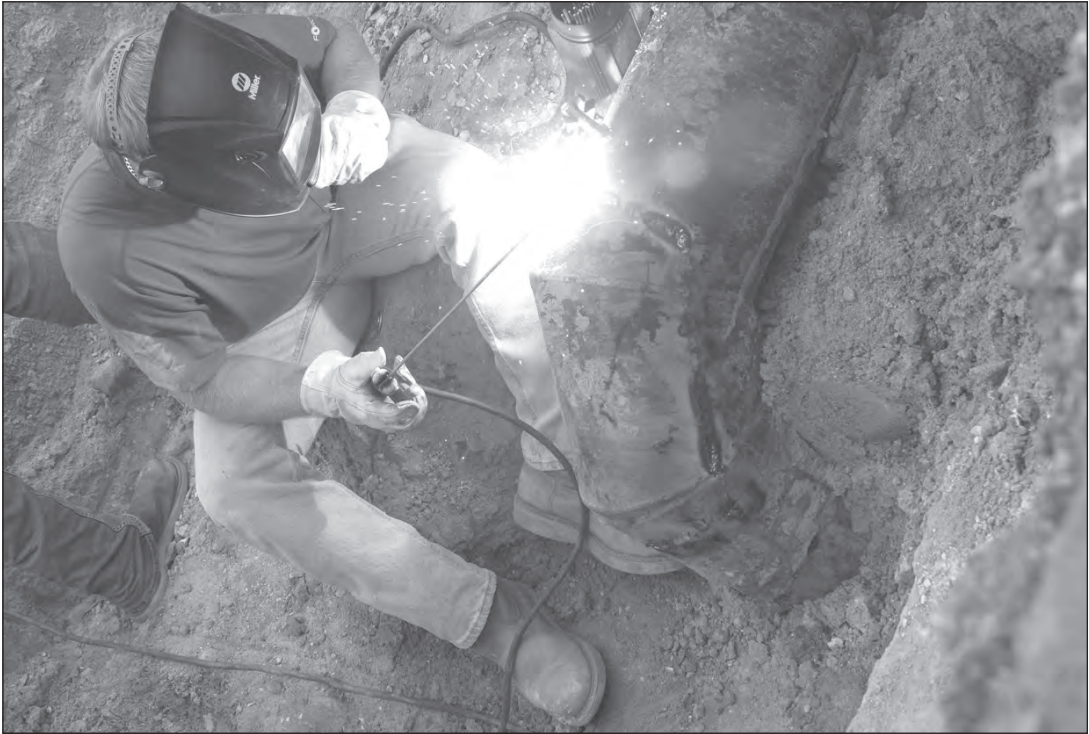
Gavin Yawn, 78th Civil Engineer Squadron industrial mechanic, welds a metal plate onto a steam vent pipe. The pipes were used for heating buildings, supplying hot water, powering industrial processes, sterilizing equipment, and regulating humidity in specialized facilities. (U.S. Air Force photo by Jerry Foltz)
