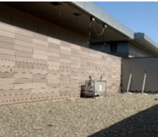
Fig. 1 - Exterior Wall Condition of Mechanical Room
