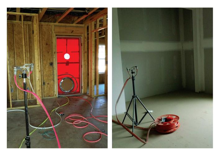
While a blower door pressurizes the house, emitter nozzles pump a fog of acrylic sealant into the building air. Walls can be exposed sheathing (above left) or finished with drywall (above right); either way, the aerosolized sealant flows out through any air leaks and coagulates on small openings as it encounters a reduction in temperature and humidity.
