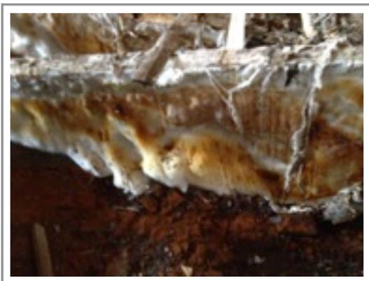
Beams & Floor Boards destroyed by rampant dry rot over large areas with floors collapsing & very dangerous
