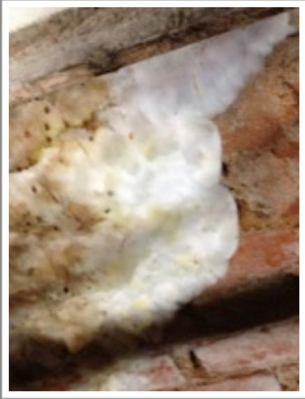
Walls substantially covered & infested with dry rot up to the window cills to date.
