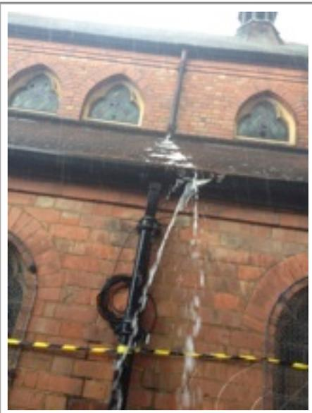
Gutters significantly blocked & wrong specification for the flow of water from these large roofs.
