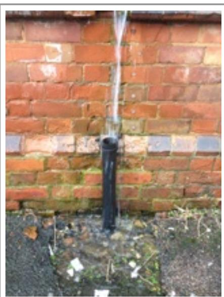
Ground level drains smashed & filled with concrete & tarmac in alley way. Water has no where to go but back in to Wesley's, which it has done for the past 30 years.
