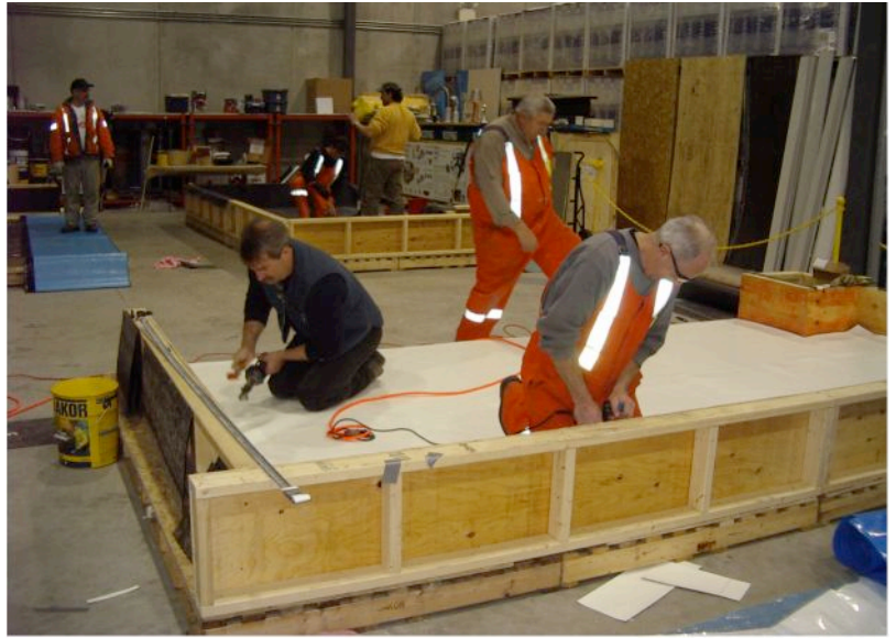
PVC deck, welding procedure for repairs.
