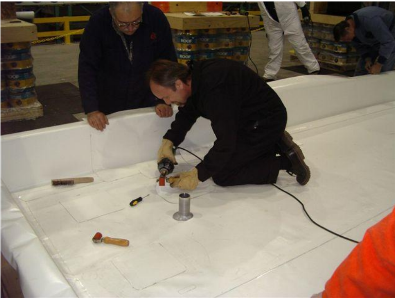
PVC Deck, Proper Welding Procedure for Repairs.
