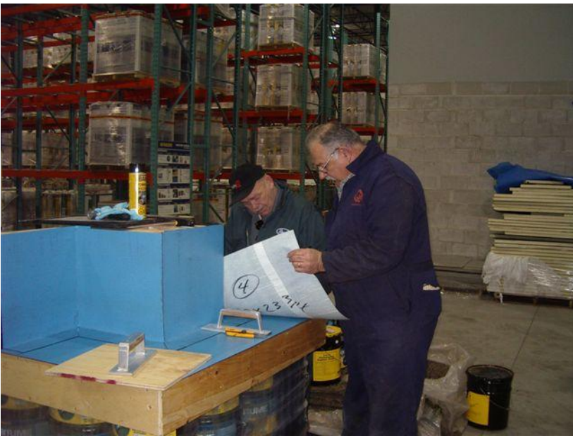
Inside & Outside Corner Detailing, 2 Ply Modified Bitumen Peel & Stick application.
