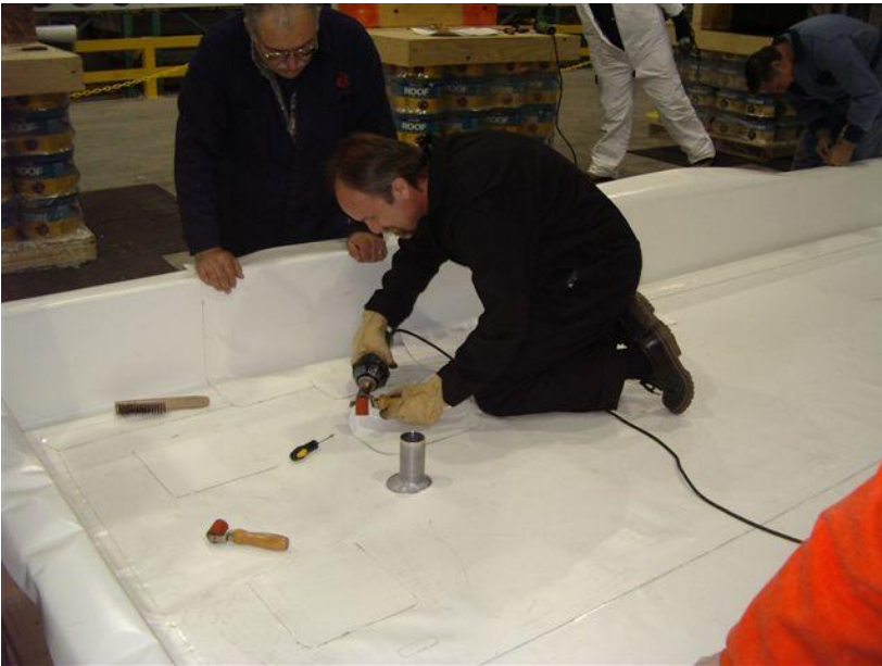
PVC Deck, Proper Welding Procedure for Repairs.
