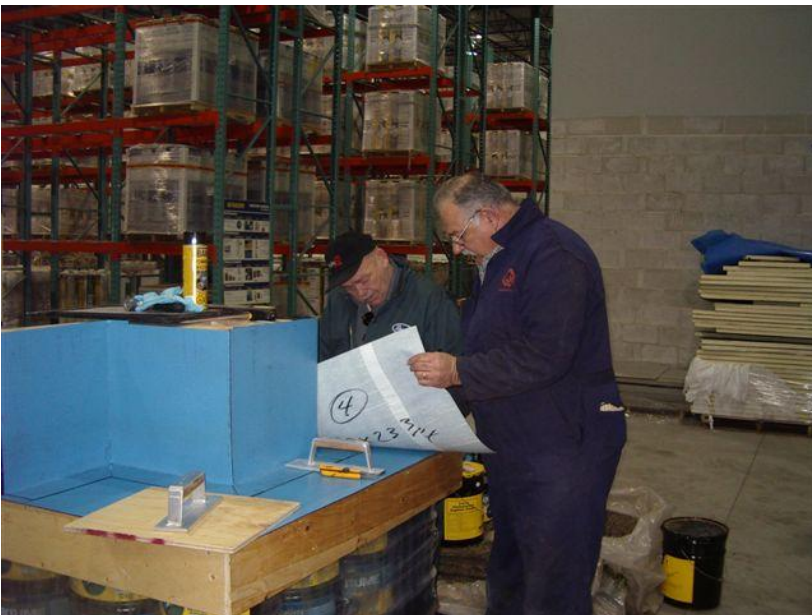
Inside & Outside Corner Detailing, 2 Ply Modified Bitumen Peel & Stick application.
