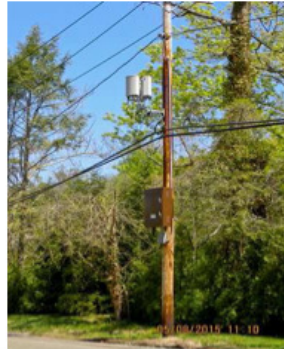
Single-carrier DAS Node on Long Island
