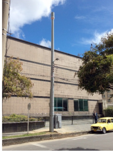
New approach: 35' Combination Utility/Light Pole/Cell Site
