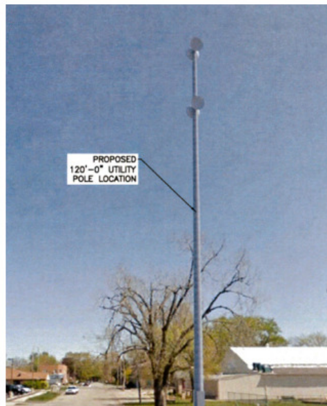
Mobilite 120' microwave backhaul facility in R-O-W
