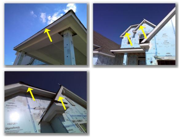
• Poorly installed flashing observed at the front and back sides of the structure.
