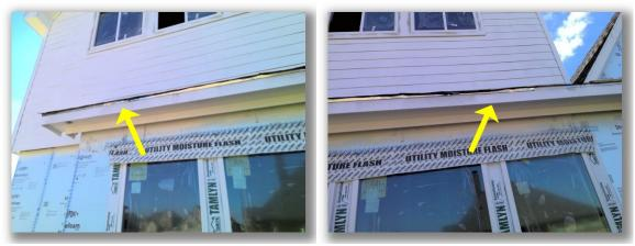
• Missing drip edge flashing observed at the front and back sides of the structure.
