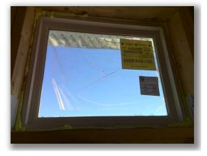
• The tape flashing is not properly installed at and around one or more of the windows on the front side of the structure above front entry door.
