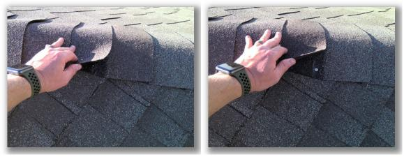
• Note: Roof fasteners (nails and/or staples) were observed to be exposed and should be properly sealed at the ridge caps and flashing areas.
