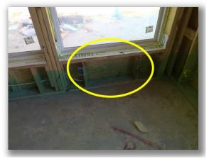
• One or more of the wall studs was observed to be bowed in the living room. This condition should be corrected prior to installing the drywall finish.
