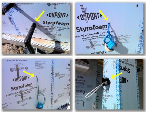
• The holes and/or openings (utility, doors, windows, etc.) in the exterior sheathing / weather barrier should be properly sealed (mastic or tape) on the right and left sides of the structure.
