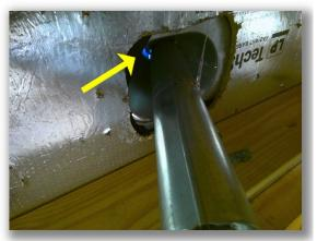
• One or more of the roof level plumbing vent stack flashing details are buckled downward around the plumbing stack. This condition could allow water penetration at this point and corrective measures are recommended.
