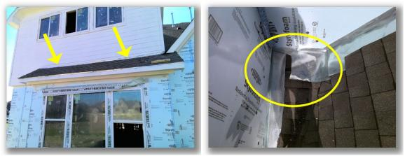
• One or more of the flashing detail flanges are not properly set into the roofing material. This condition needs to be corrected to help prevent water intrusion at this points.
