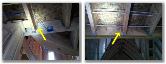
• One or more joist hanger(s) do not have enough fasteners (nails) installed in the under under stairway closet.
