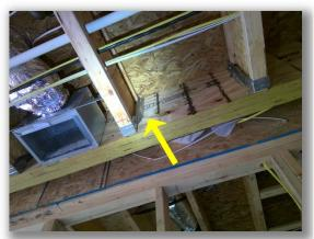
• One or more joist hanger(s) do not have enough fasteners (nails) installed in the kitchen.
