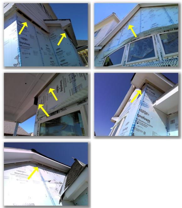
• There is no visible through wall "head" flashing details install above the exterior doors on the front and back sides of the structure. Under current building standards, through wall "head" flashing is required to be installed to help prevent water intrusion from occurring at this point.
