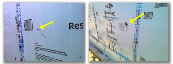
• The over driven nails in the exterior sheathing / weather barrier should be properly sealed (mastic or tape) on the above front garage area of the structure.
