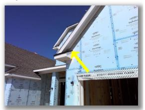
• There are not enough veneer ties "brick-ties" in place on various locations of the structure. Under current building standards, each tie shall support not more than 2.67 square feet of wall area and shall be spaced not more than 32 inches on center horizontally and 24 inches on center vertically.
