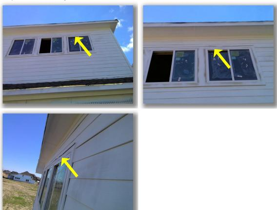
Poorly installed Z flashing observed over the windows in att the back of the structure.
