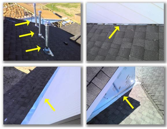
• Recommend painting all metal flashing & flues to help prevent rust/deterioration.
