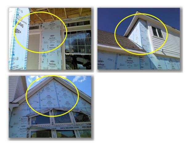
Missing sheathing and/or blocking observed at the front and back sides of the structure.
