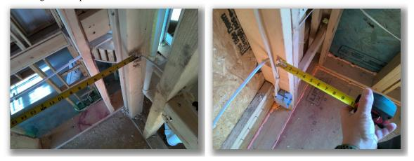
• The electrical junction box does not properly set out 1/2-inch from the wall stud in the gameroom.
