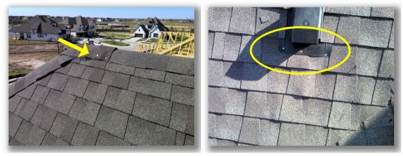
• A toe board was observed to be nailed to the shingles at the back side of the structure. Recommend removing the toe board and repairing any damaged shingles.
