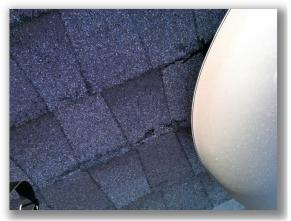
• Poorly adhered ridge cap shingles observed at the back side of the roof structure.
