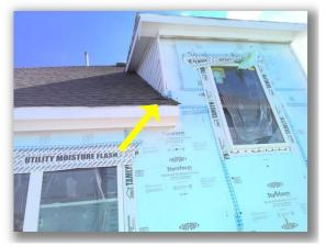
• The storm collar(s) at the roof level gas equipment vent pipe(s) need to be properly sealed to help prevent water intrusion into the structure.
