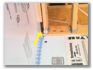
• One or more joist hanger(s) do not have enough fasteners (nails) installed in the laundry room.
