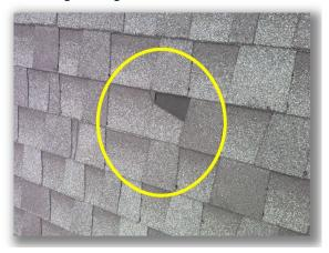
• Damaged shingles were observed on the back side of the roof structure.
