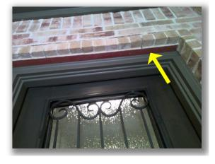
• Note: Minor mortar and/or brick cracks were observed in the exterior veneer on the right side of the structure.
