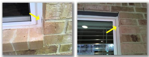
• The wall expansion joint(s) need to be properly sealed on thefFront of structure/outside front door of the structure. It is recommended to use an elastomeric caulking.
