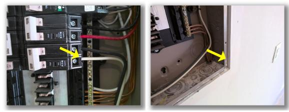
• The breakers (overcurrent devices) in the electrical panel are not properly labeled.
