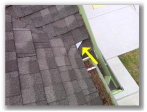
• The storm collar(s) at the roof level gas equipment vent pipe(s) need to be properly sealed to help prevent water intrusion into the structure.
