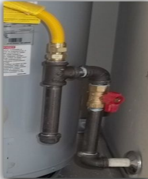
Samples of correct sediment trap installations
