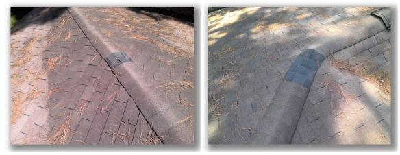
• Algae and/or an organic growth on the roof covering is an indication that the roof is older and may be near the end of its expected serviceable life. Recommend consulting a roofing contractor about the possibility of cleaning and or replacement in the near future.
