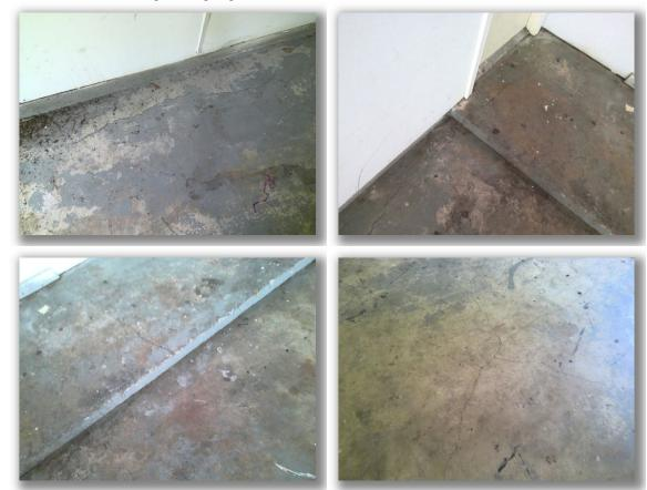
• Note: Some cracking of the garage concrete floor finish was observed.
