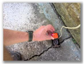
• One or more of the receptacles appear to have reversed polarity (i.e. it is wired backwards). This receptacle(s) and the circuit should be investigated and improved as necessary. The receptacle(s) in question are located in the living room.
