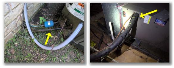
• The electrical wire conduit has pulled loose at the outside condenser housing and/or service disconnect.
