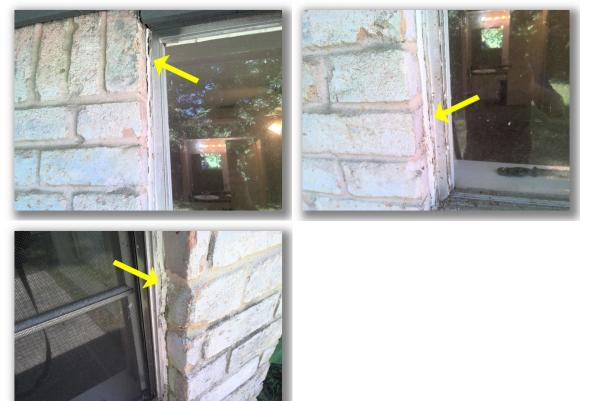
• Caulking improvements are recommended for the area between the exterior veneer and the garage door trim boards. It is recommended to use an elastomeric caulking.
