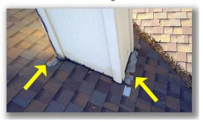
• One or more of the flashing detail flanges are not properly set into the roofing material. This condition needs to be corrected to help prevent water intrusion at this points.
