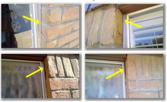
• The area between the exterior cladding / veneer and all of the wall penetrations / openings need to be properly sealed. Areas such as utility connections, downspouts, hose bibbs, lighting fixtures, receptacles etc. It is recommended to use an elastomeric caulking / sealant.
