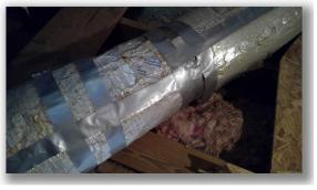
• The duct work in the attic area does not appear to be properly suspended and separated to help prevent condensation form developing. It is recommended to separate and suspend the duct work with supports in minimum intervals of 4-feet that have a minimum width of 1.5-inches.
