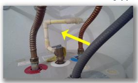
• There is no pan installed under the water heater.
