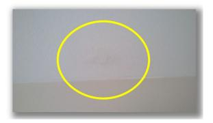
Note: Nail heads were observed to be pushing through the interior finish in one or more locations.
