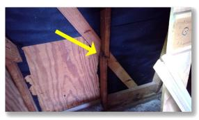
Interior wall stress cracks were observed in the master bedroom.
