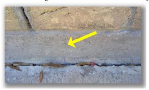
• One or more of the post tension cable ends are exposed and need to be properly sealed on the right side of the detached garage.
