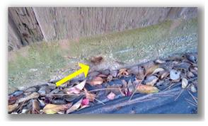
• Note: Tree(s) in close proximity of the foundation was observed. Client should consider the installation of a root barrier to reduce the possibility of damage to the foundation from tree roots and moisture removal.
