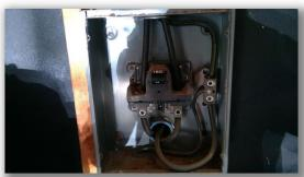
The electrical cabinet cover plate (dead front) should be installed with blunt tip screws and not sharp wood type screws for reasons of safety.
