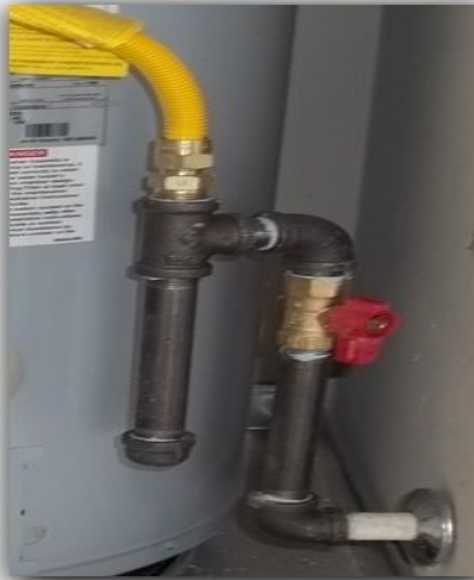
Samples of correct sediment trap installations
