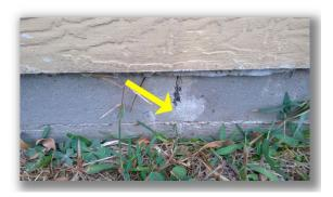
One or more of the post tension cable ends are exposed and need to be properly sealed on the back side of the structure.
