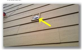
One or more of the mechanical exhaust vent systems was observed to be terminating to the soffit / eave area. This is an "AS Built" condition that does not meet current manufacturers or mechanical installation standards.
