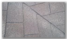
• Damaged shingles were observed on the back side of the roof structure.
