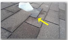
Some of the metal flashing details were observed to be rusted and should be corrected as necessary.
