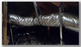
• Some of the ductwork in the attic area has been turned to sharply. This will restrict the airflow through the duct system and affect the airflow balance in some areas of the house.
