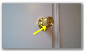
Door handles to hall bathroom and rear corner bedroom have damaged/sharp metal edges.
