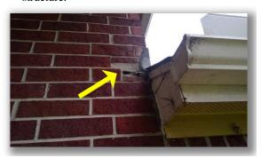
Caulking improvements are recommended for the area between the exterior veneer and the window frames. It is recommended to use an elastomeric caulking.
