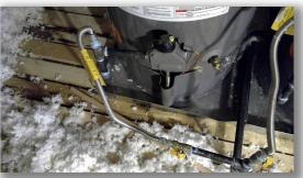
The water heater flue connector should be mechanically attached to the draft hood with a minimum of three sheet metal screws.
