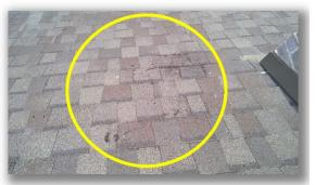
• Damaged shingles were observed on the southeast of the roof structure.
