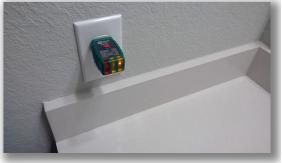
• One or more of the receptacles were observed to have an open neutral connection in the master bathroom.
