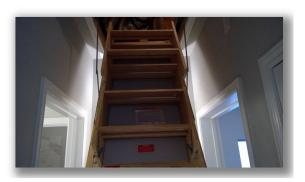
• Some of the attic ladder nuts and bolts were observed to be loose and/or missing. Minor improvements to the attic ladder are recommended for reasons of safety. \*\*\*Pull down bolt\*\*\*
