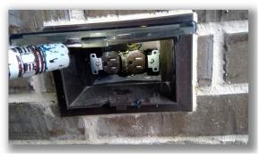
• One or more of the receptacles were observed to have an open neutral connection in the Jack and Jill bathroom.
