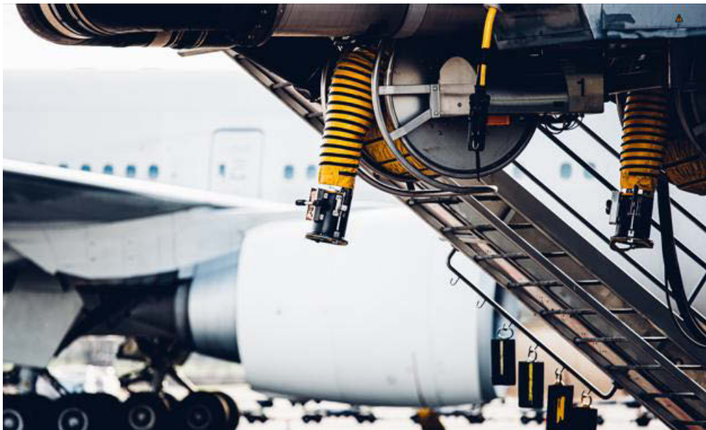
FIGURE 2-9 Example of a PCA hose reel. SOURCE: iStock.com/Fabian Gysel.
