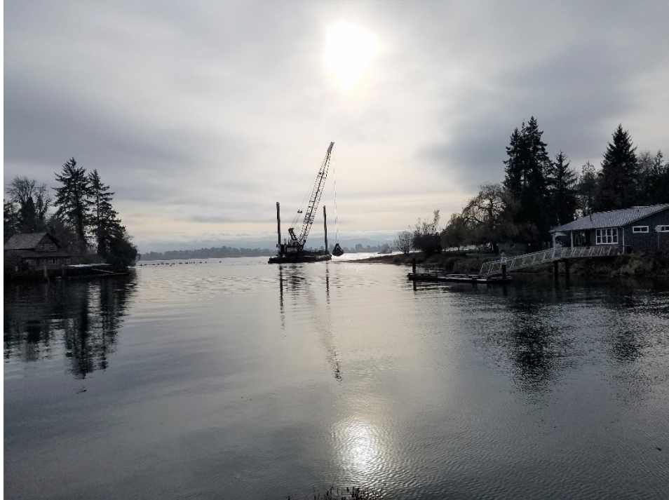
Dredging the Skamokawa Creek Entrance
