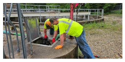
Shawn and Luke were able to pump the sludge tank at the downtown sewer plant using our old pump truck. This tank catches the non-dissolvable materials from the system before it enters the Biosolids tank. The material was then taken back to headworks and put through the
