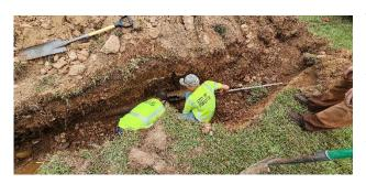
There were several tense days as utility contractors preformed work along Coy Avenue. The guys marked the water lines associated with the corner of Coy and Allen only to discover that our city maps were wrong and that the 6" main water line was not where it was supposed to be. The
