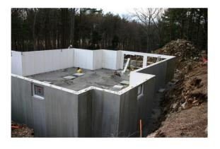
The foundation walls were precast from 7000 psi concrete, Cleantech says.
