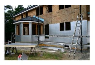
Walls were insulated with closed-cell foam on the inside and, on the exterior, foam board.
