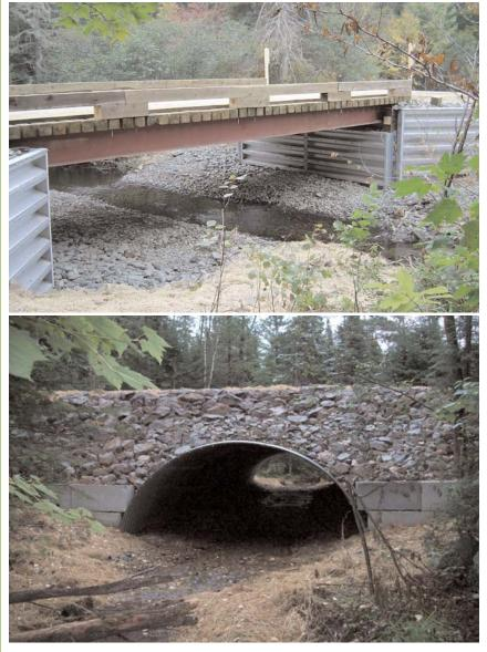
**Top - Steel stringer bridge with bolt-a-bin abutments.** (Photo courtesy of Fornebu Lumber) **Bottom - Multi-plate open bottom arch.** (Photo courtesy of AV group)
