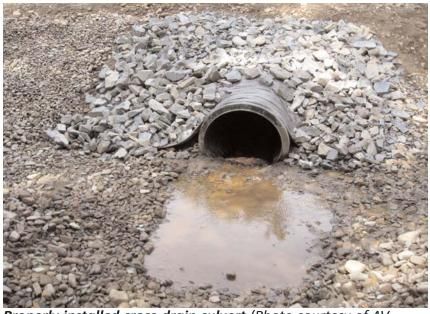
**Properly installed cross-drain culvert** (Photo courtesy of AV group)
