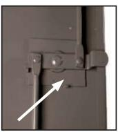
1/8" thick latch and 3/8" diameter lock rods
