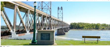
It was originally built in 1924 and was the first permanent bridge crossing the Missouri River. This unique bridge is a "double-decker" with one lane positioned above another and a lift-span to allow riverboat traffic to traverse the river. Up until 1953, it was operated as a toll bridge. In 2015 the Meridian Bridge Plaza was added to the north end of the bridge and is now home to a fountain, splash pad, benches, shading, green space, Yankton Riverwalk (sculpture trail)
