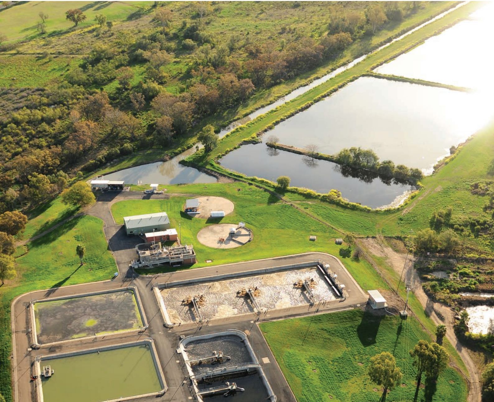
Moree Sewerage Treatment Plant
