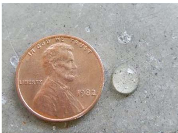
FIG. 1 Non-absorptive Concrete Surface
