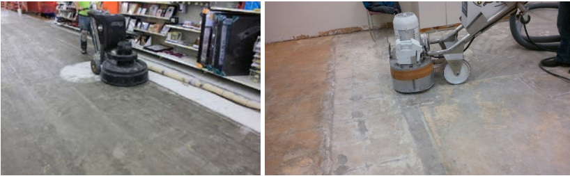
Example of floor grinders w/ shrouds + dust control
