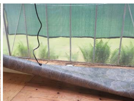
Then the linoleum was laid out. We are not carpenters or experienced floor people so we picked a single piece of linoleum.
