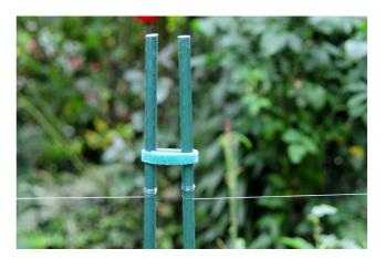
Fig 4. Close-up of poles at one side of a Gate to the garden. Gate is Temporarily Held Closed with Removable Velcro Loop. The Fence is Made Using Stren Lo-Vis Green 12 lb. Fishing Line strung on 6 ft x 5/8 in Green Garden Stakes.
