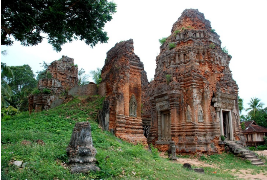
Lolei – Picture of the old conditions of the temple, around 1998-2000 with the towers in degraded conditions to the south covered by earth and grass. They were in perilous conditions and the Apsara Authority made simple wood supports to the doors with lintel and forbid the entrance to the internal ones (Photo Damien & Okh 2000).
