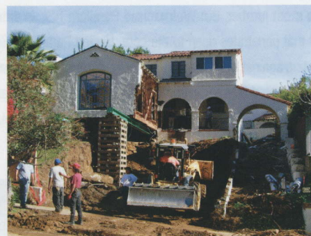
Ashland: This home had to be supported on temporary steel beams so that construction could go on below and beside the house.
