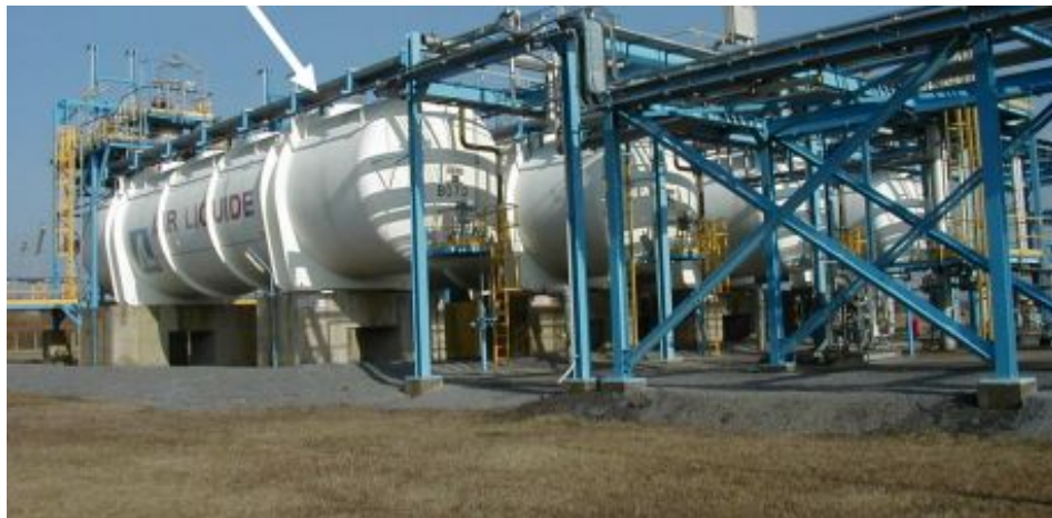
LH 2 storage tanks at Waziers liquefaction plant in France (10 t.d -1 )
