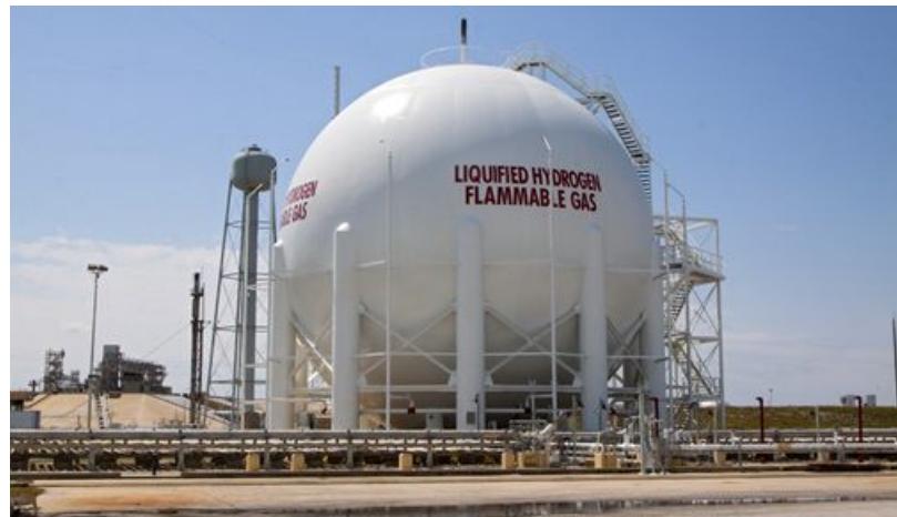
LH 2 storage vessel with 3 800 m 3 capacity at KSC in Florida
