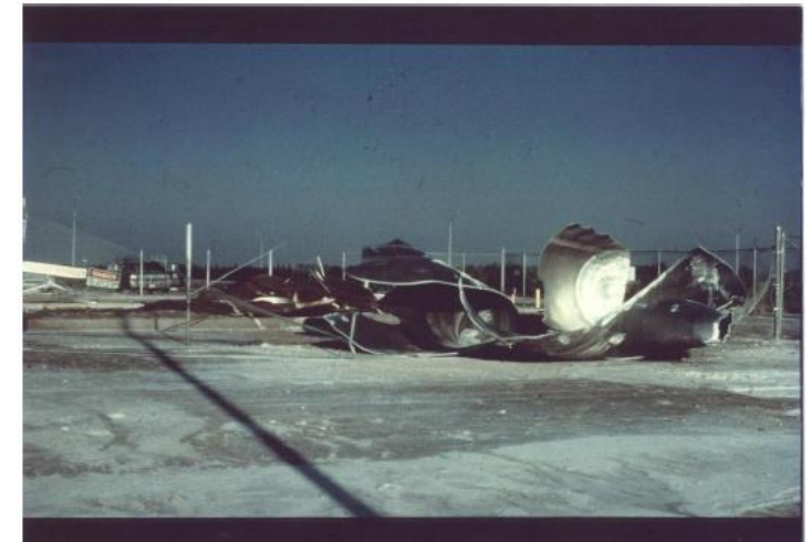
Catastrophic rupture of a 76 m 3 \text{LH}_2 storage tank (Shen and Miller, 2024).
