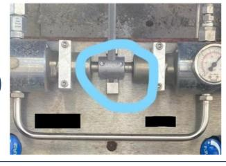
Before taking any action, check which ramp is actually in service using the arrow on the selector
