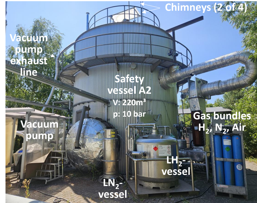
Outside view of safety vessel A2 during the Fire Tests
