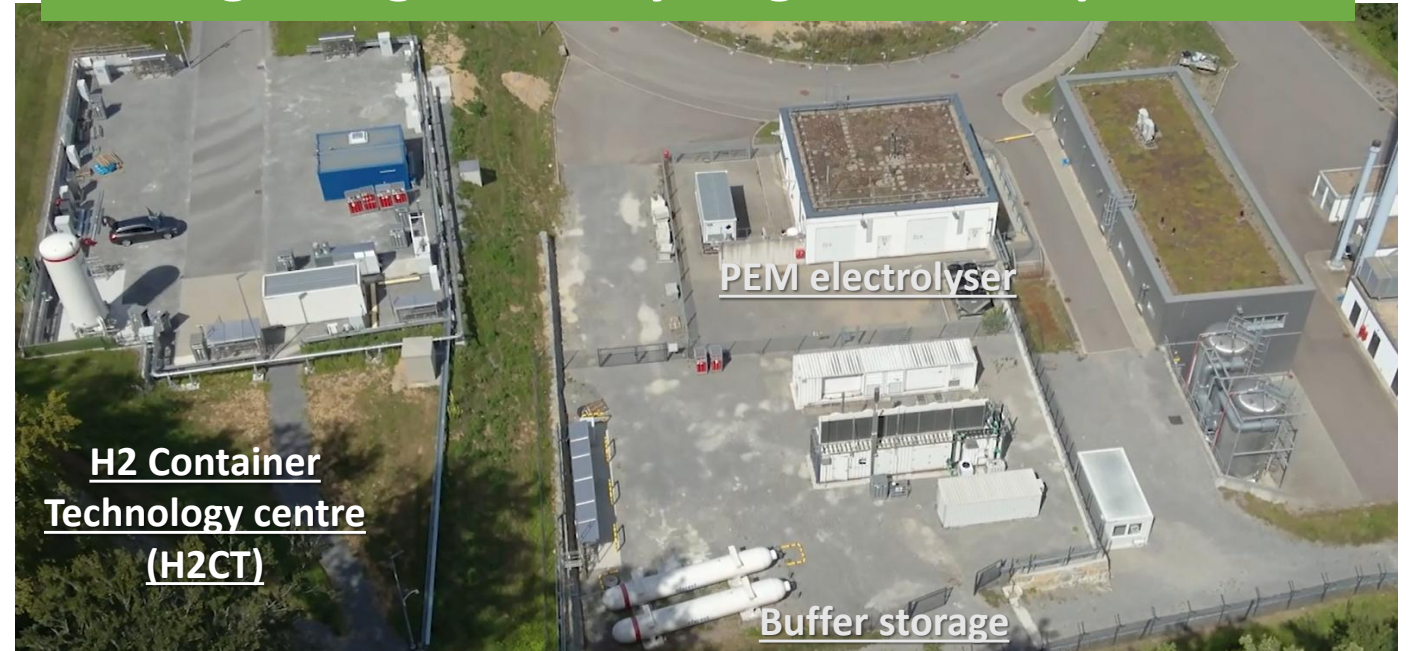
100% green gaseous hydrogen on-site produced
