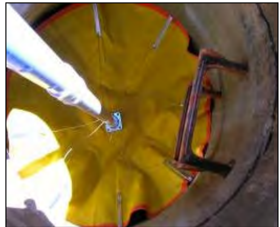
Debris Dam Placed in Manhole
