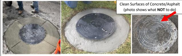
Note: Many other products and methods that can be used to reduce infiltration and provide other benefits. This guideline is intended to represent the optimum method for installing utility access covers. The life and performance of any access cover depends on proper installation.
