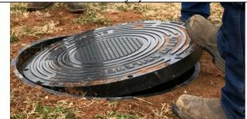
You may need to rotate the cover if the holes and hardware do not line up. The frame has shapes (triangles, stars) that indicate where the bolt holes should be aligned to have the cover and frame holes centered on each other. The frame also has indicators for paddle lock notches.
