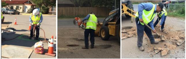
4) Inspect the access hole opening and remove any dirt, grease or other debris from the access hole opening and support.
