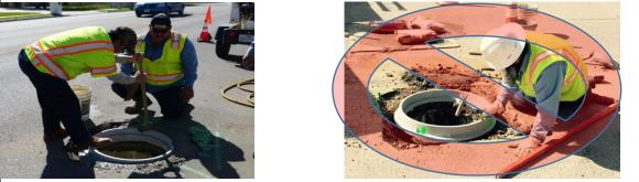
13) Holes in the frame flange can be used to anchor with bolts into the riser rings or concrete below. This is not mandatory, but the holes in the frames allow for this option. (See end of instructions)
