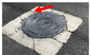
Note: Improper install can reduce product life and voids warranty. Municipalities are responsible for training contractors on correct installation procedures. Applying the surrounding concrete too shallow could cause cracks and expose the frame edges to side impact. Frame edges should be flush or slightly below grade – Areas with freezing will need to determine the depth below grade to allow for ice heaving.
