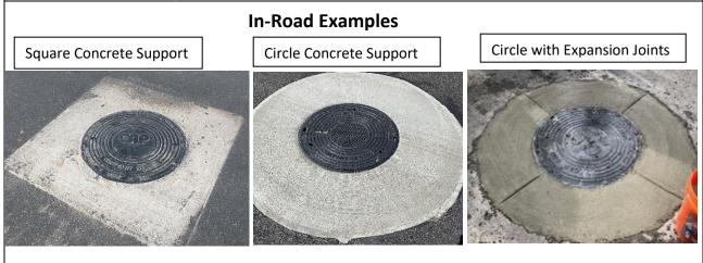
Note: Off-road some will simply backfill with dirt, raise with concrete to avoid lawnmower impact, or raise several feet to prevent water inflow.
