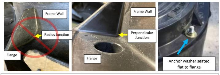
CAP frame flanges are perpendicular to the vertical frame wall. This allows for a washer to sit flat under the nut on the threaded rod used for anchoring the assembly. Non-perpendicular (radiused) flange-wall junctions can tilt the washer with one side propped up on the vertical wall joint.
