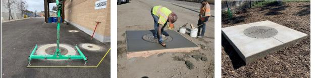
Note: If tripod use is planned for entering and exiting the manhole, it is adviseable to have a solid supporting surface large enough for the tripod base. Tripods may not be secure on dirt or soft ground. Some municipalities specify 12 feet by 12 feet of concrete around manholes.
