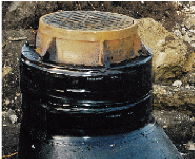
High shrink membrane conforms to irregular structures.
